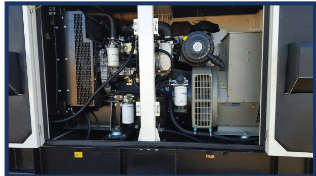
EASY ACCESS FOR MAINTENANCE
